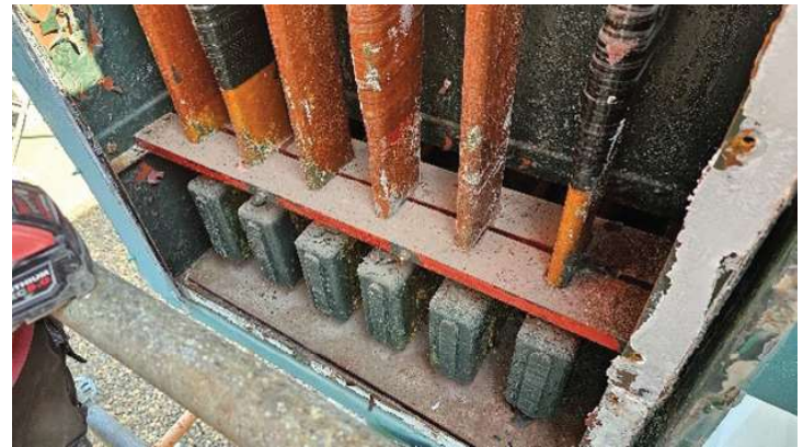
Old Failing Bus Work
