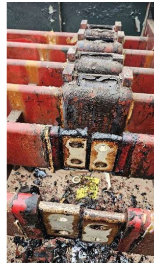
Old Failing Bus Work
